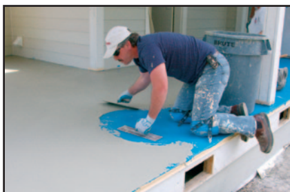
KRETE KOTE/TOP COAT BEING APPLIED
