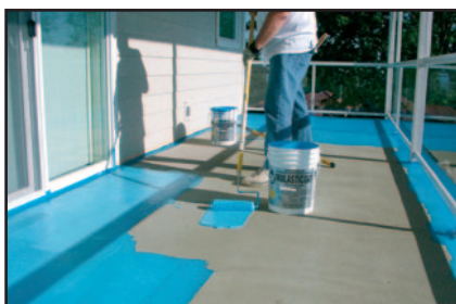
APPLY TWO COATS OF MULASTICOAT, "THE BLUE STUFF"
