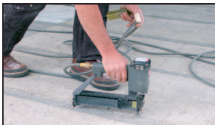
STAPLE METAL LATHE TO DECK
