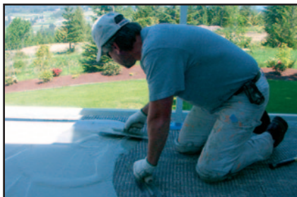
MULTI-BASE APPLIED, COVERING METAL LATHE
