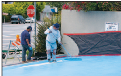
WATERPROOFING ENTIRE SURFACE WITH MULASTICOAT
