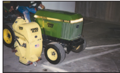
SURFACE PREP (SHOT BLAST)
