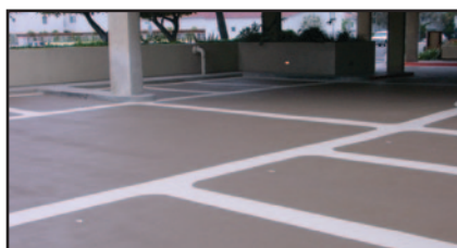
ALLOW TO DRY MIN. 48-72 HOURS BEFORE OPENING TO TRAFFIC
