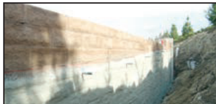
SECOND COAT - MULASTICOAT - ROLLED OR SPRAYED
