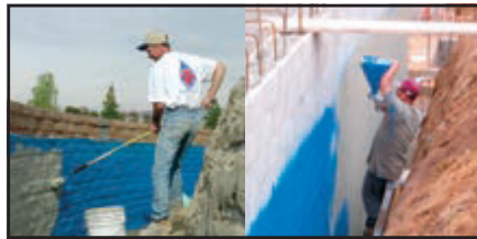
FIRST COAT - MULASTICOAT - ROLLER OR SPRAY APPLIED
