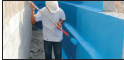
Second Coat - "The Blue Stuff" Roller or Spray Applied
