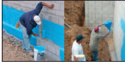
First Coat - "The Blue Stuff" Roller or Spray Applied
