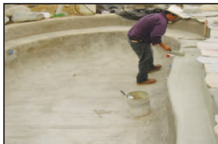
INITIAL SCRATCH KOTE 2000 APPLICATION
